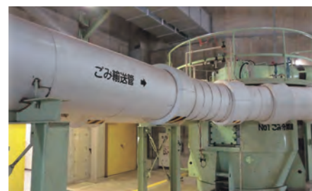
廃棄物空気輸送管 Pneumatic trash-carrying ducts
